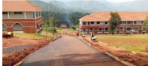
Roads under construction
